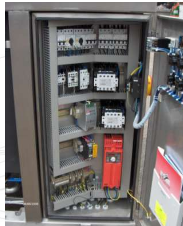
Mobile mixingtanks, Pick & Place unit.
